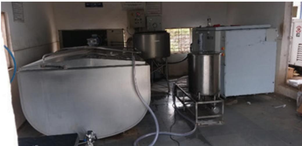
Figure 35: Bulk Milk Cooler
